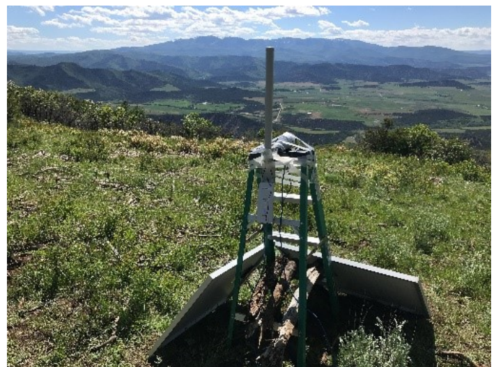
Figure 1—Mountaintop Radio Site During Test Deployment
